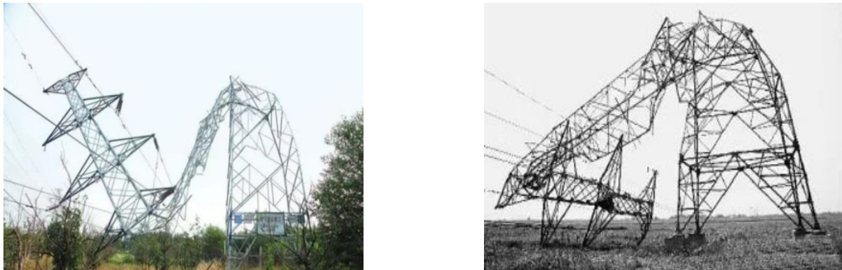
Figure 1. Collapses of transmission towers under downburst winds.
